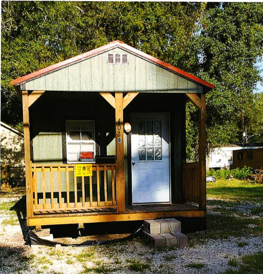
Portable Building, facing Washington Ave.
