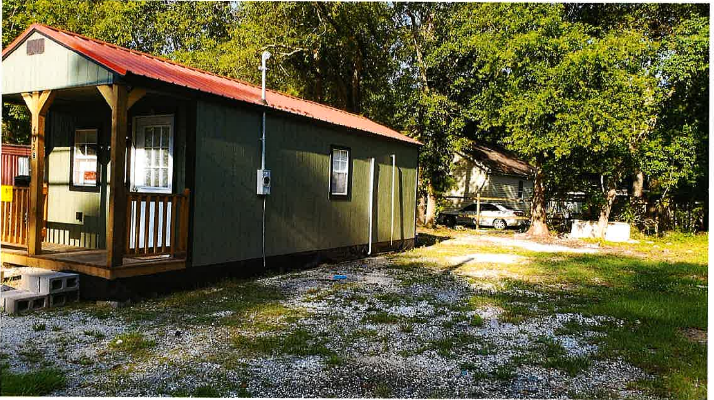
North side of Portable Building
