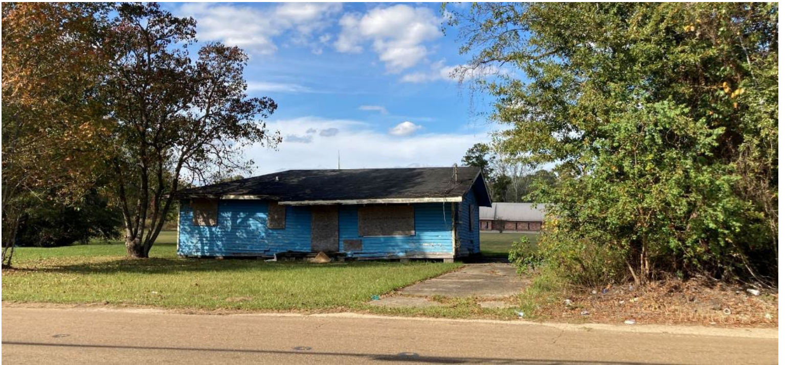
Facing North of 706 Magazine – across street
