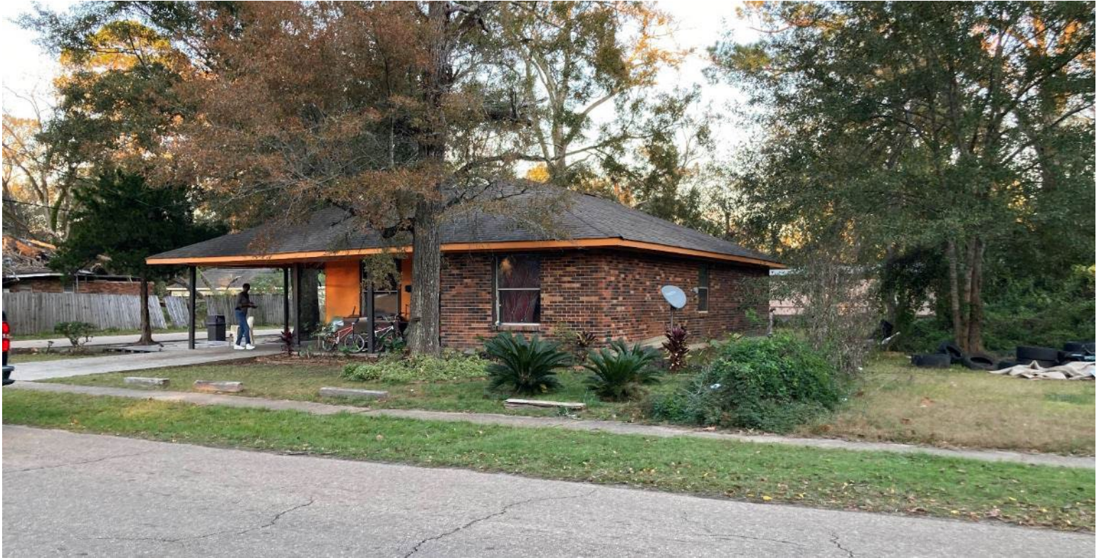
Facing east – across street – Single-family home
