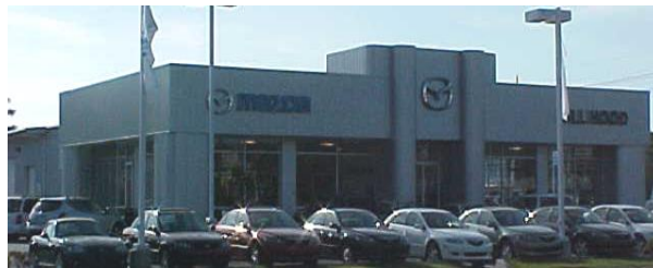
(Example of an acceptable metal building)
