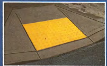
HIGH PRESSURE WASHDOWN TO CLEAN ADA RAMPS
