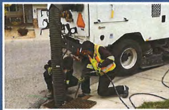
CATCH BASIN CLEANING OF DEBRIS AND POLLUTANTS
