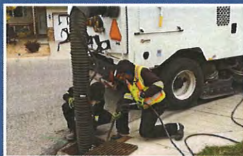
CATCH BASIN CLEANING OF DEBRIS AND POLLUTANTS
